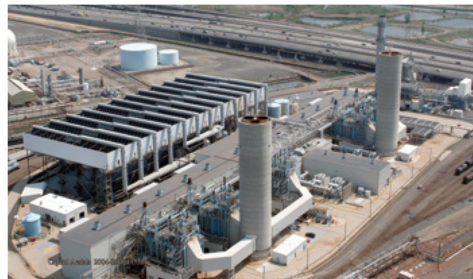
Hydrogen Power-enabled Linden Gas Thermal Power Station Unit 6 (US)
